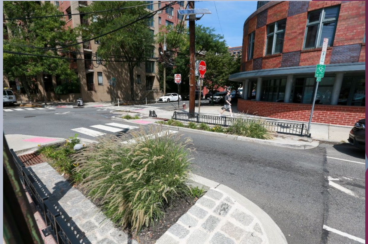
Example of stormwater bump-outs in Hoboken, NJ.
